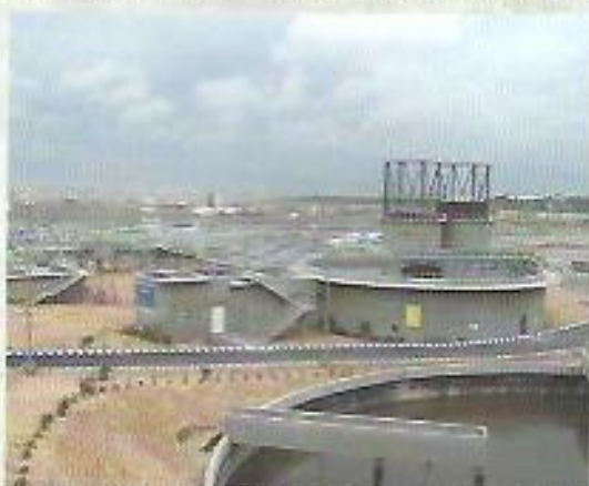
A view of Combined Effluent Treatment Plant (CETP) Korangi Karachi.
