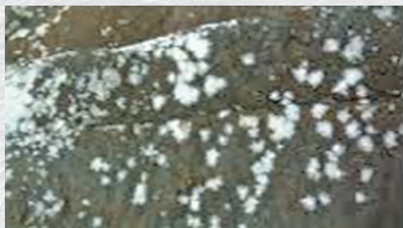
Fatty Spew (Major Defective Area)
